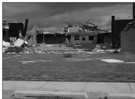
The aftermath of the 2004 Norris tornado.
